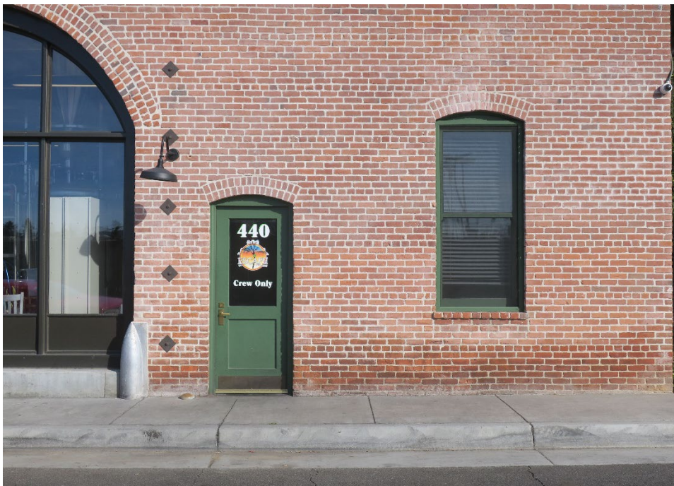
Photo 6 Close-up view of the south façade new/restored door opening and window opening.
