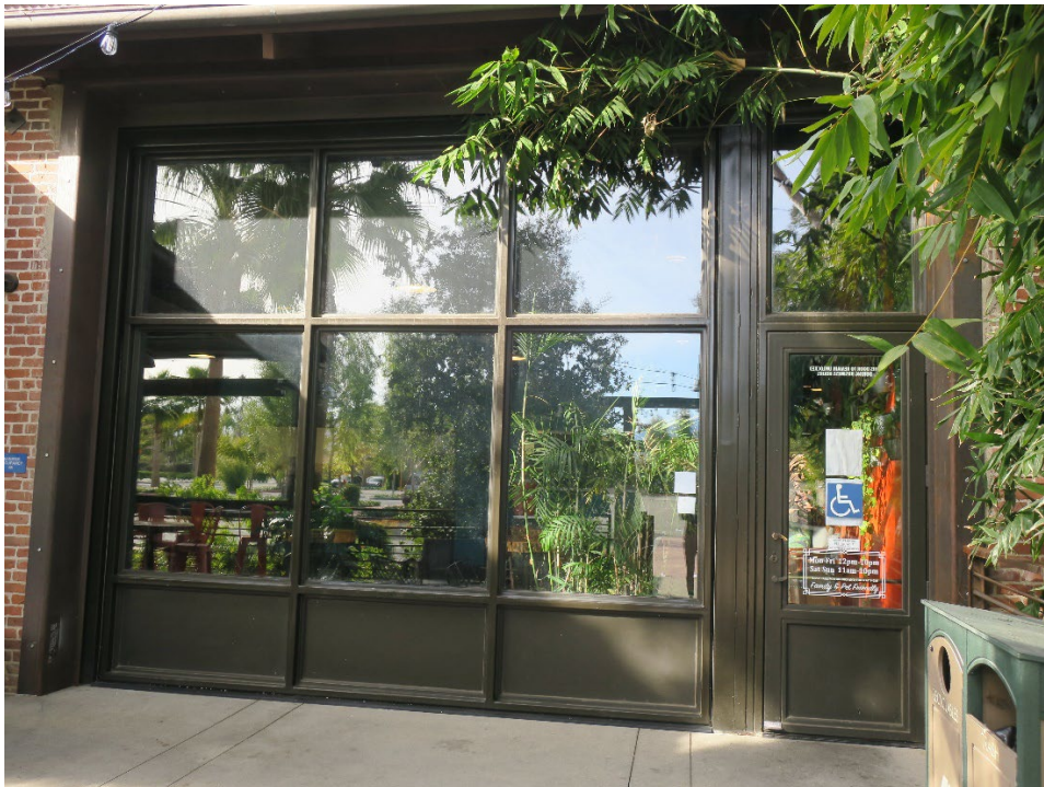
Photo 12 Close-up of the new tilt-up steel door assembly at the north end of the east façade.
