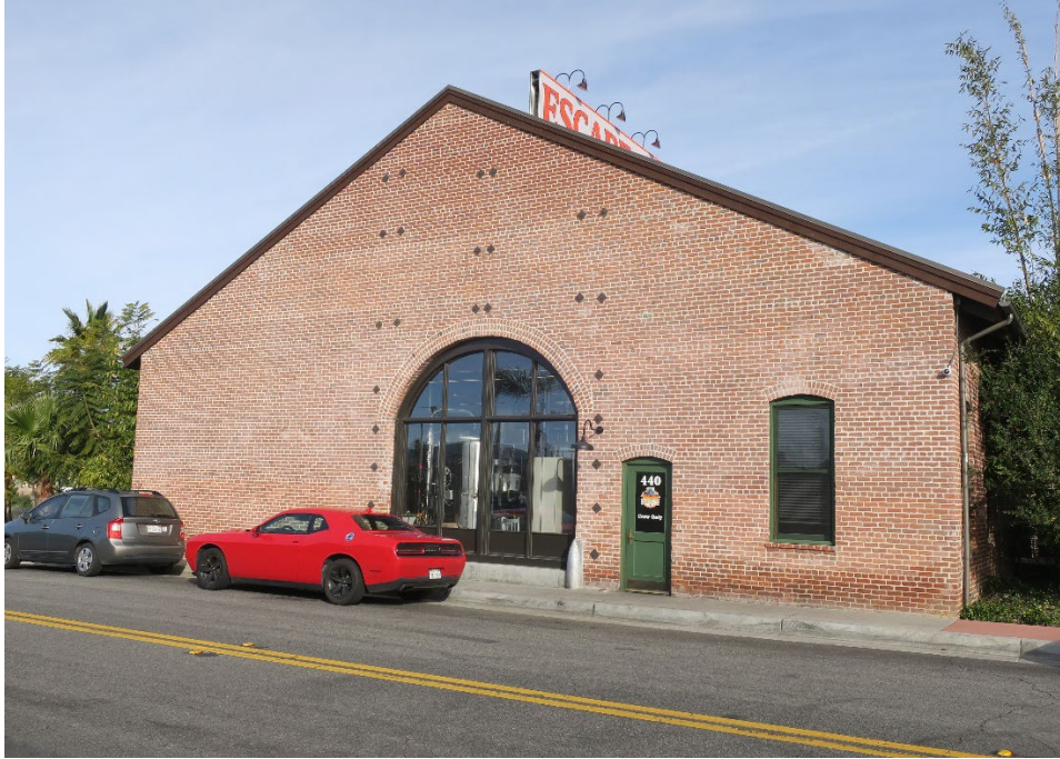
Photo 6 Close-up view of the south façade new/restored door opening and window opening.
